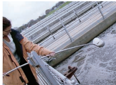
A wastewater treatment plant.
